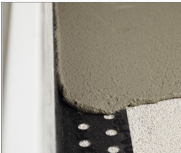
Figure 6 Application of plaster
