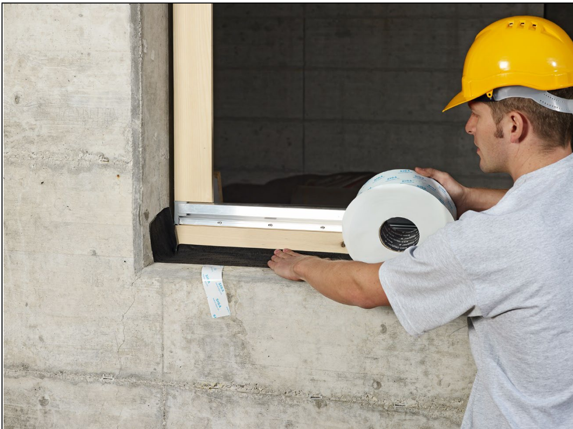
Figure 3 Installing tape at bottom of frame
