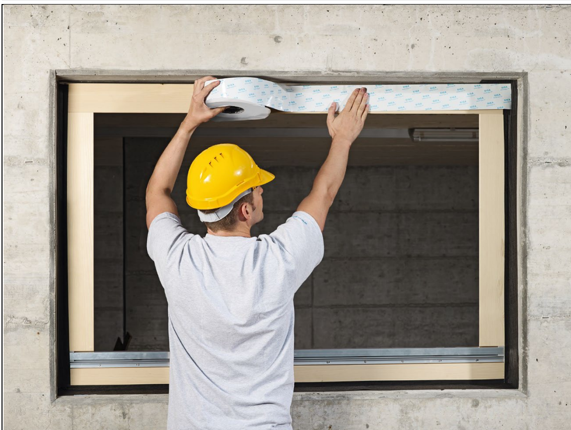
Figure 5 Installing tape at top of frame
