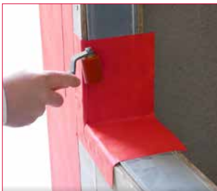
Fig.06: Use roller to ensure proper adhesion of Wraptite Corners to substrate.
